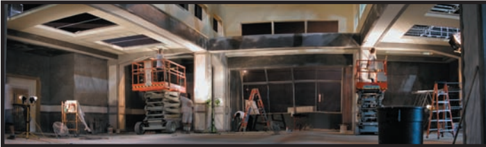
“CAFFETERIA” SET UNDER CONSTRUCTION
